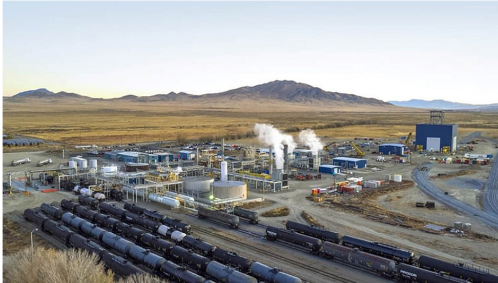
Figure 1. Cyanco Facility in Winnemucca, Nevada (Credit: Cyanco)
