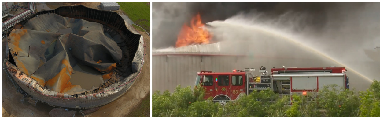
Figure 13. Post-incident photo of the damaged tank (left, Credit: IMTT) and the emergency response to the tank fire (right, Credit: WWL-TV).
