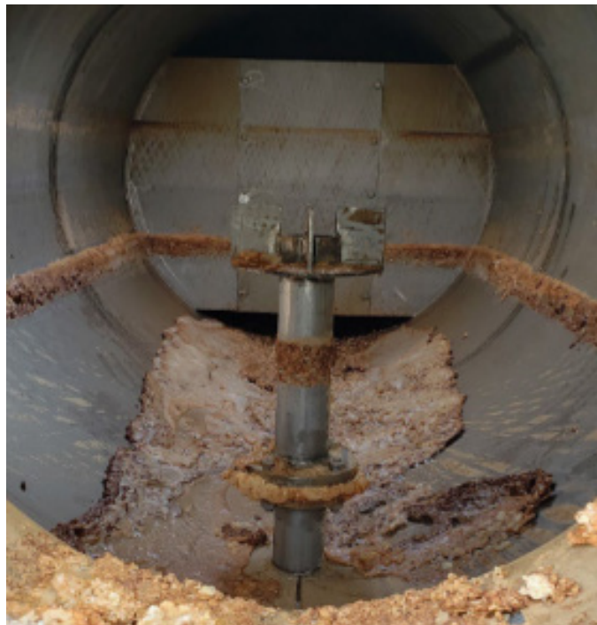
Figure 1. Tank Containing Solids at SABIC. (Credit: SABIC)
