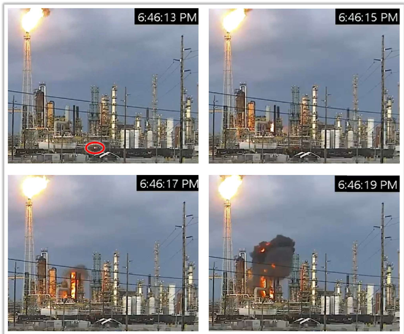
Figure 11: Vapor cloud ignition and the ensuing six seconds. Ignition at Crude Furnace (circled in red, upper left photo). (Credit: BP with annotations by CSB)
