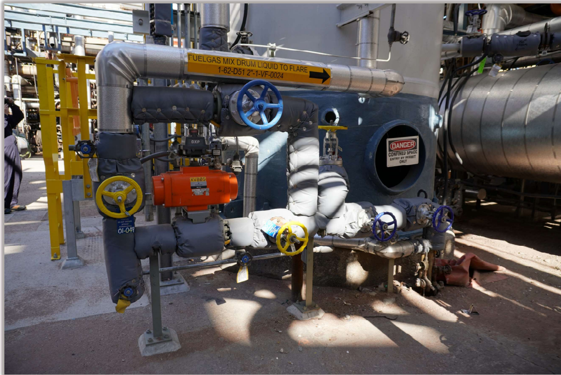
Figure 32. Toledo Refinery Fuel Gas Mix Drum with modifications made after the September 20, 2022, incident. (Credit: CSB)
