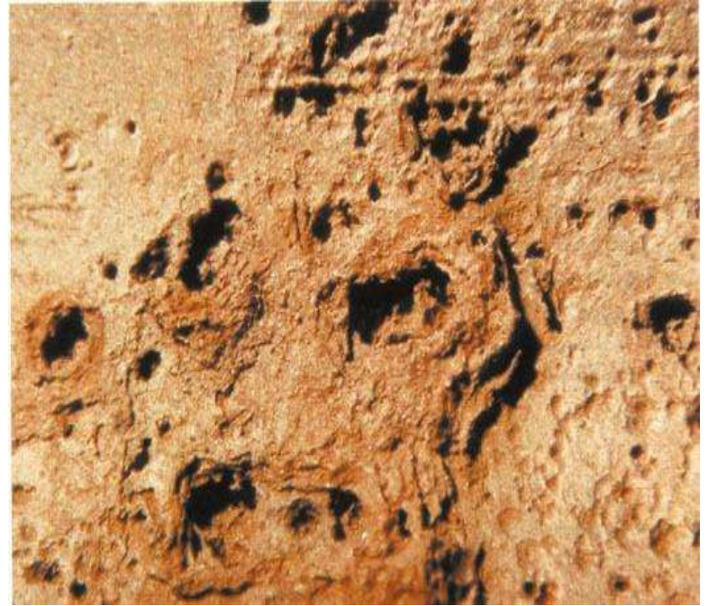
Deposits on turbine before cleaning
