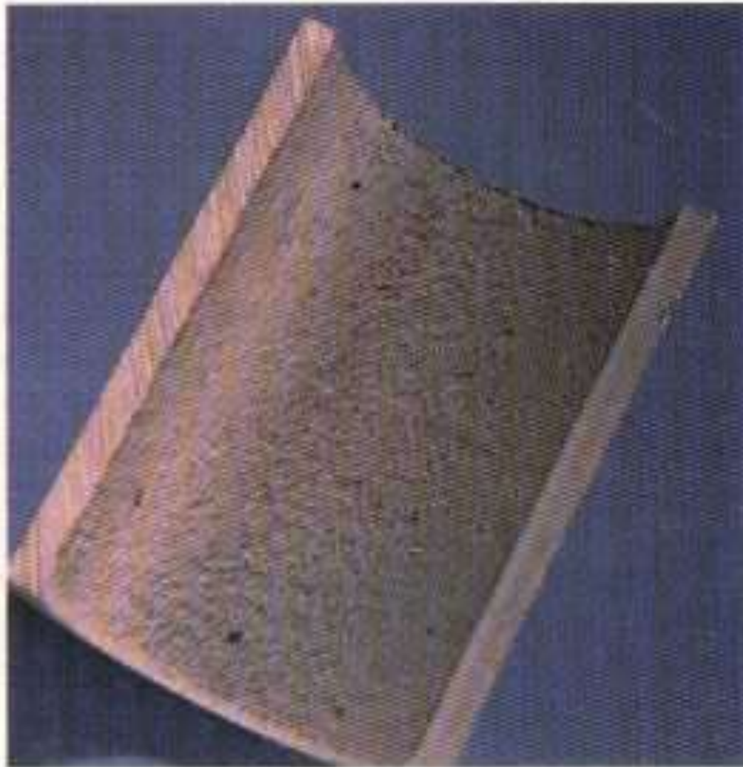
Boiler tube shows effect of acid attack.
