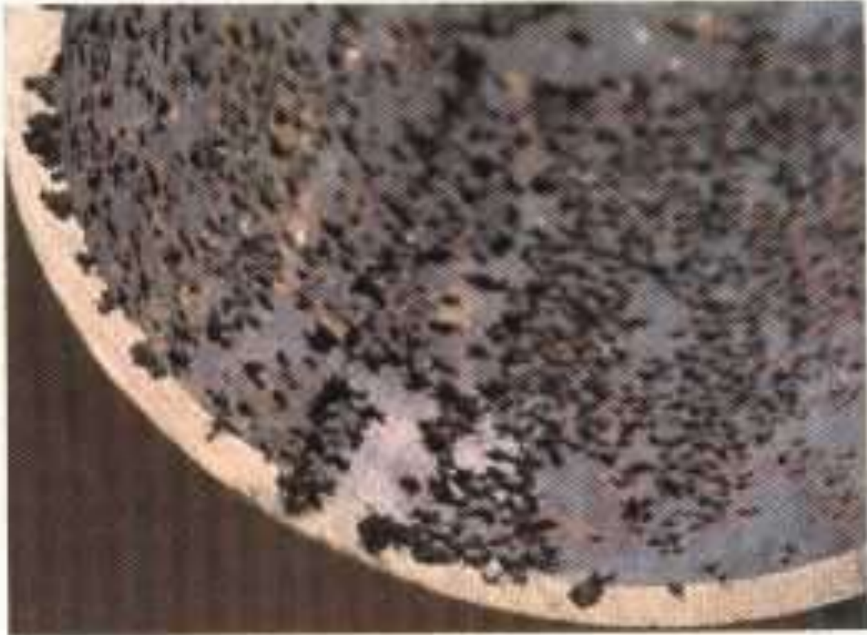
Oxygen pitting of a boiler feedwater pipe.
